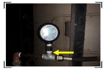
All weld joints, mechanical joints, screwed or flange, etc., should be exposed for examination during the hydro test
