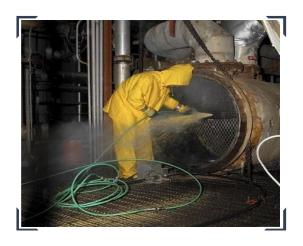
After cooling and opening all manholes, mudholes, and handholes, the vessel should be cleaned by flushing with treated water to free it from dirt, **scale**, debris, and other foreign material.
